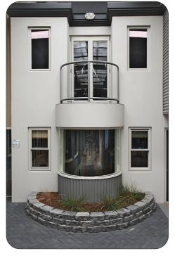
Some of the tell tale signs... Missing flashings over windows, missing flashings on parapets, garden in direct contact with cladding and penetrations through cladding to fix handrails.
